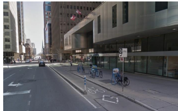
Figure 72: Example of existing separated bike lanes with pre-cast concrete curbs on Laurier Avenue, Ottawa Source: WSP Canada
