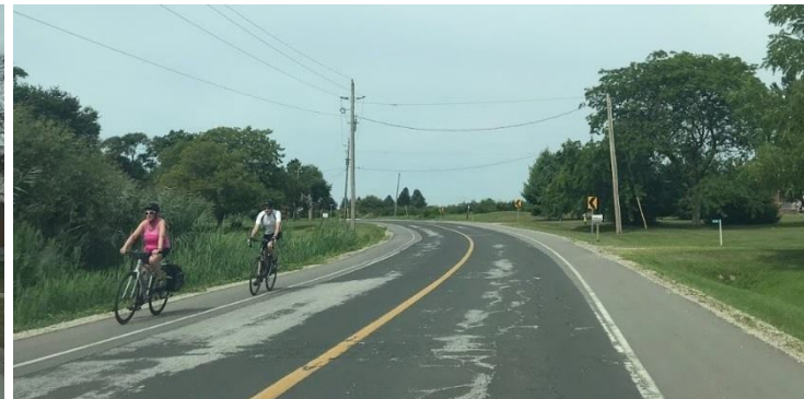
Figure 68: Existing paved shoulder on County Road 50, Essex Source: WSP Canada
