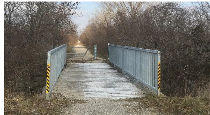
Figure 78: Existing Chrysler Canada Greenway at County Road 18, Essex Source: WSP Canada
