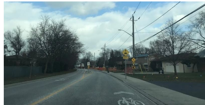
Figure 66: Existing signed route on County Road 21, Lakeshore Source: WSP Canada
