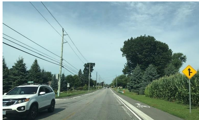
Figure 73: Existing one-way cycle track on County Road 20, Leamington / Kingsville Source: WSP Canada
