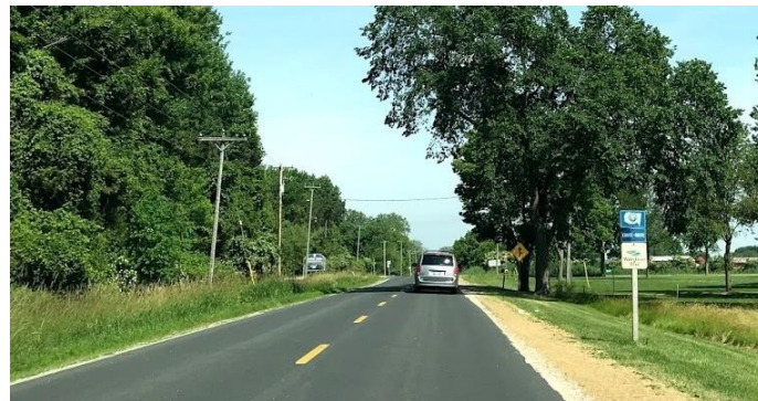
Figure 65: Existing signed route on County Road 50, Amherstburg Source: WSP Canada
