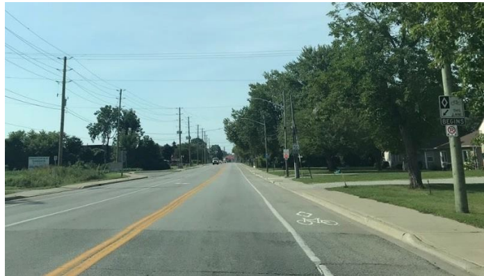
Figure 69: Existing bike lanes on Erie Street North, Leamington Source: WSP Canada
