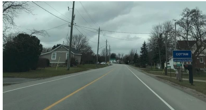
Figure 67: Existing paved shoulder on County Road 34, Kingsville Source: WSP Canada
