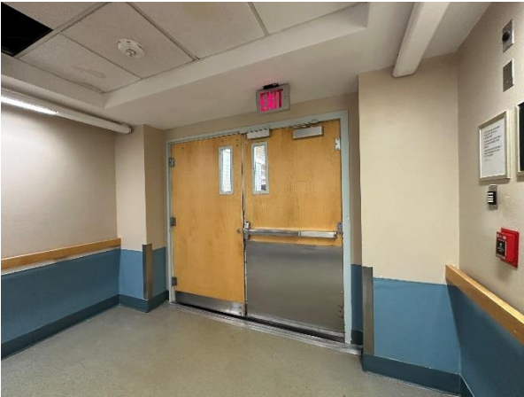
Photograph No. 23 Typical interior wood doors.
