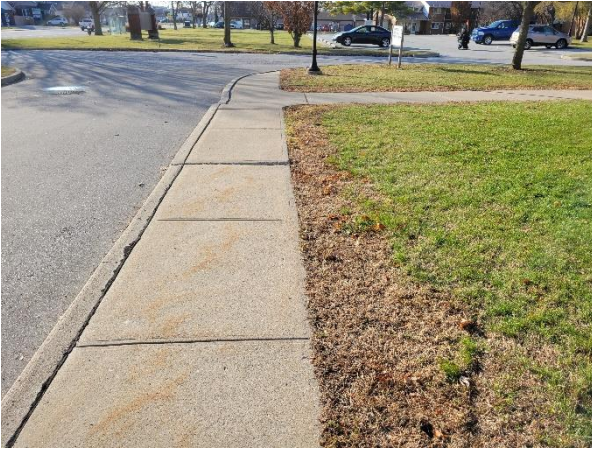
Photograph No. 65 Walkways are generally in good condition.
