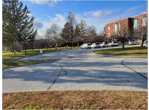
Photograph No. 66 The south drive aisle is in fair condition with surface deterioration noted throughout.
