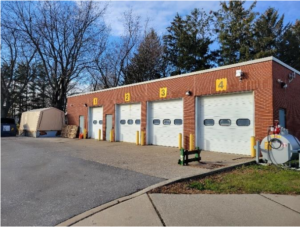
Photograph No. 21 Overhead garage doors are in good condition.
