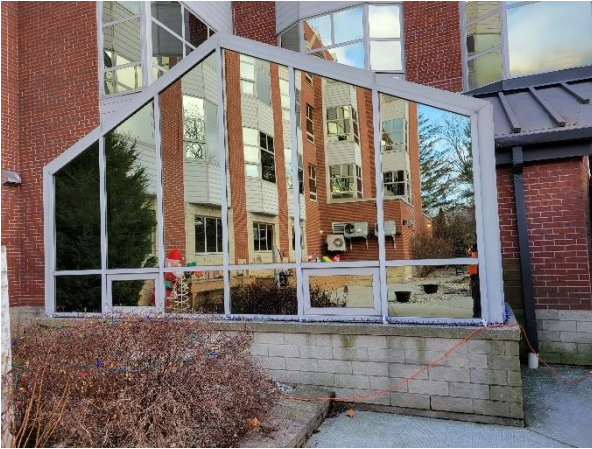
Photograph No. 13 Windows frames are generally in good condition.
