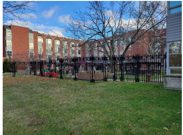
Photograph No. 4 North Elevation
