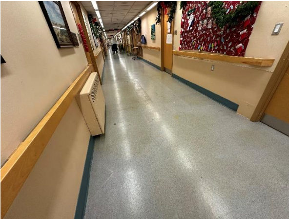
Photograph No. 35 South wing corridor finishes are generally in fair condition.
