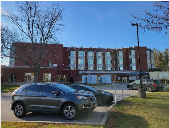
Photograph No. 3 Partial East Elevation
