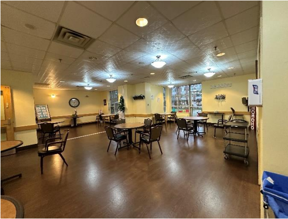
Photograph No. 25 Typical dining room finishes are in good condition.
