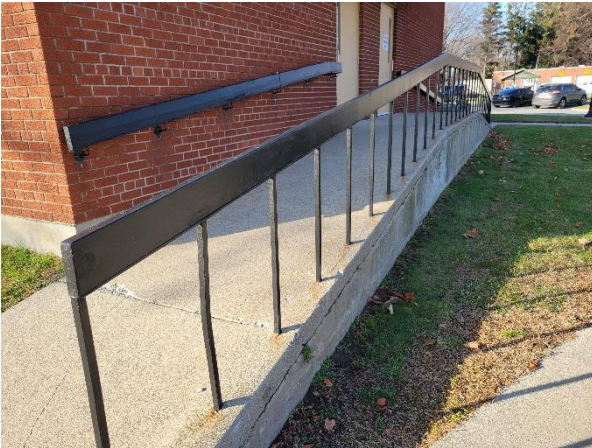
Photograph No. 71 South wing exit ramp is in good condition.
