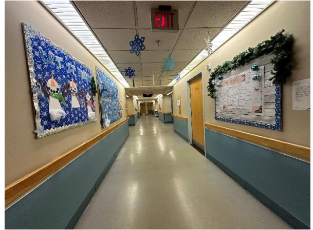
Photograph No. 26 Typical corridor finishes are in good condition.
