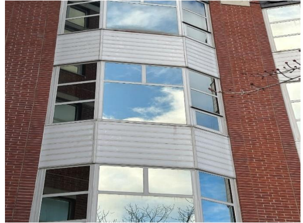
Photograph No. 14 Typical window wall and metal siding configuration.
