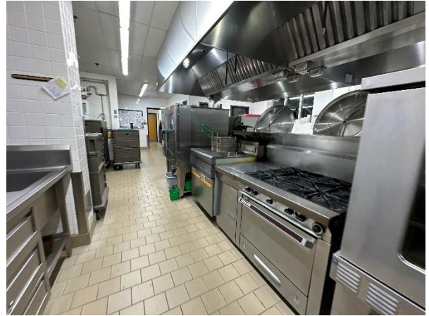
Photograph No. 34 Kitchen finishes and appliances are generally in good condition.
