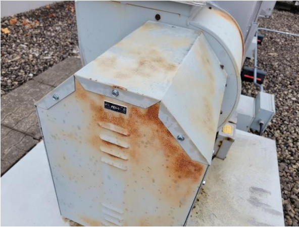
Photograph No. 45 Rooftop exhaust fans are original but appear to be operational.
