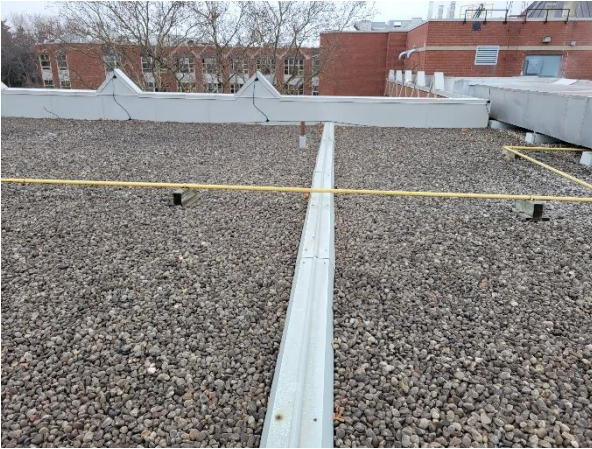
Photograph No. 17 Expansion joint in inverted roofing system at main roof.
