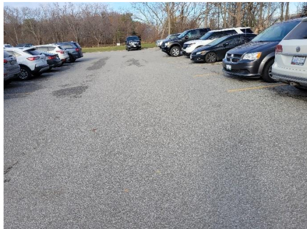
Photograph No. 64 Paved asphalt parking areas are in good condition.
