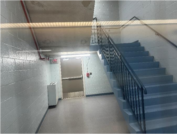
Photograph No. 29 Typical stairwell finishes are in good condition.
