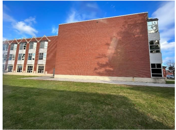
Photograph No. 2 Partial West Elevation
