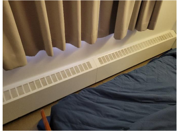
Photograph No. 58 Radiators throughout are generally in good condition.
