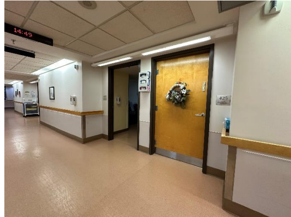
Photograph No. 38 Solid wood resident room doors.
