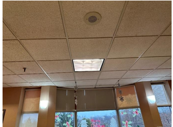
Photograph No. 32 Drop ceiling finishes are generally in good condition.
