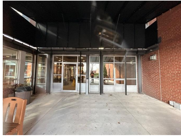
Photograph No. 22 Glazed entrance doors are in good condition.
