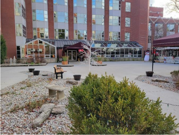
Photograph No. 69 Rear concrete surfaces are generally in good condition.
