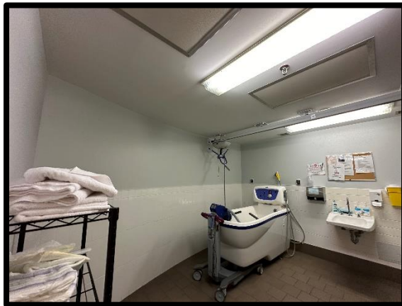
Photo 5: Typical resident bathroom with radiant ceiling.
