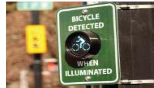
Figure 81: Bicycle Detection Indicator
